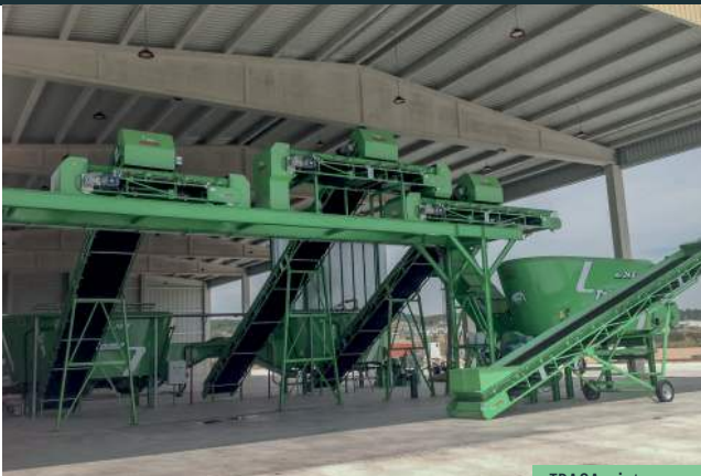
TRASA, vista general
